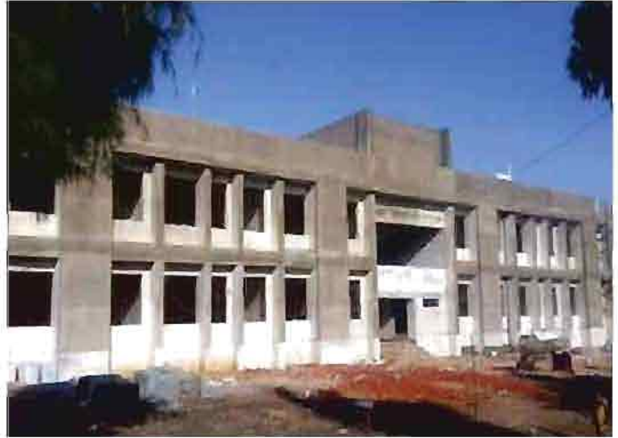
Under Construction School at Tarapur Village in Gujarat
