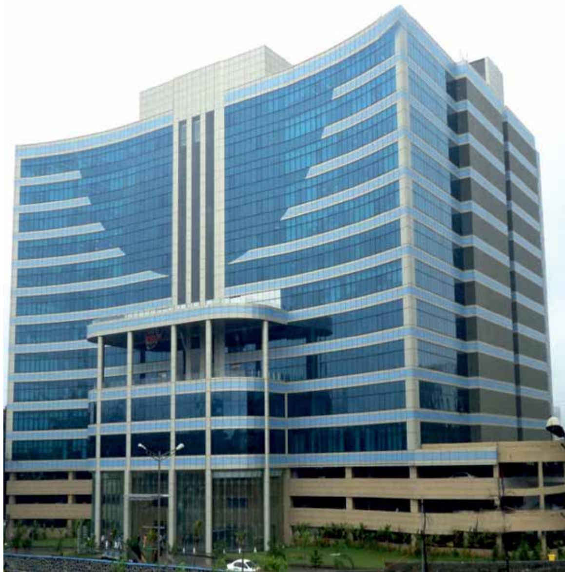
IT Building No. 3
